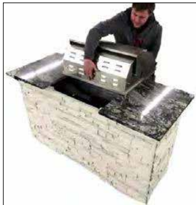
Placing the Grill Head
