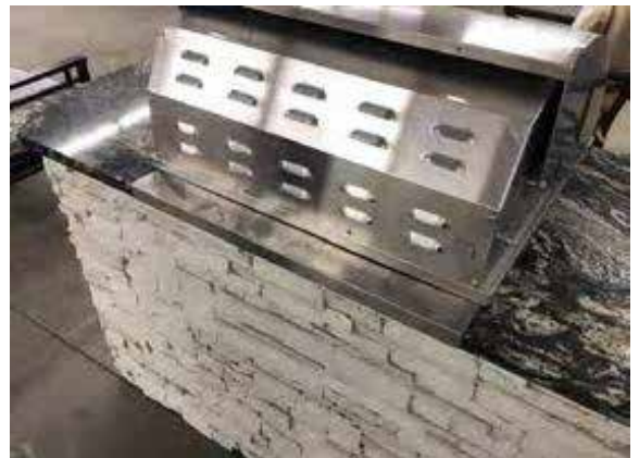
View behind the Island after Grill Head is placed
