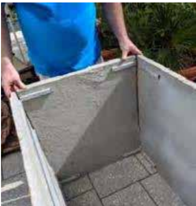
Assembling the Frame
